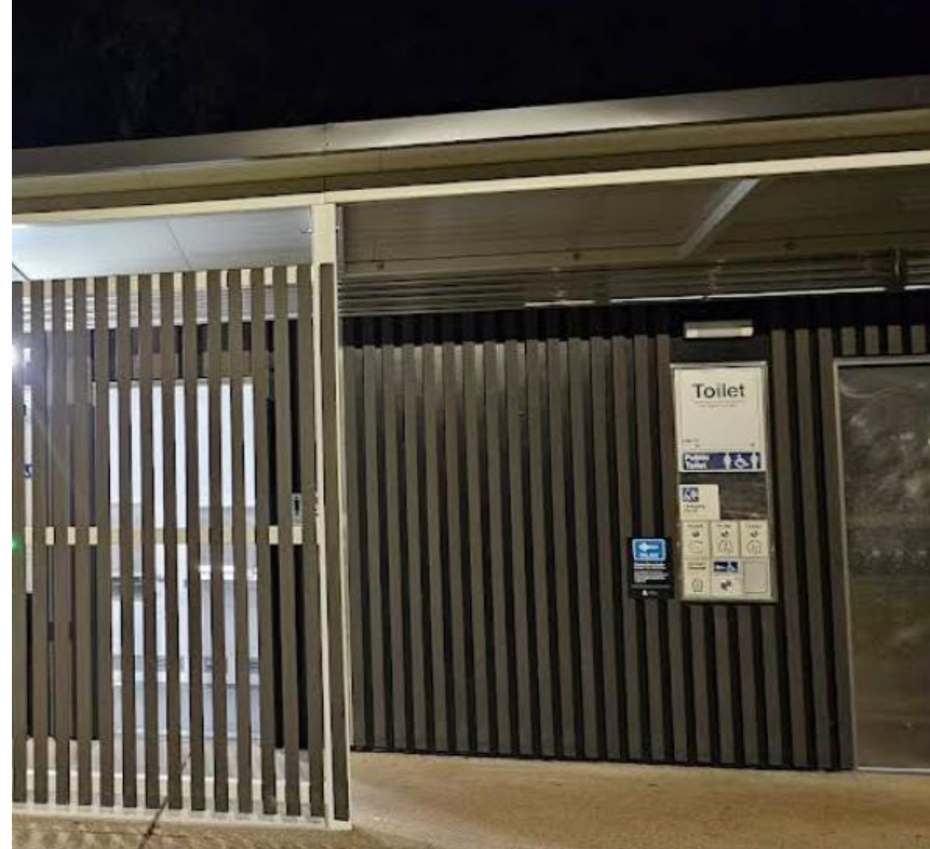
Alt Text: Rymill Park Public Toilet and Changing Places facility is visible with signage.
