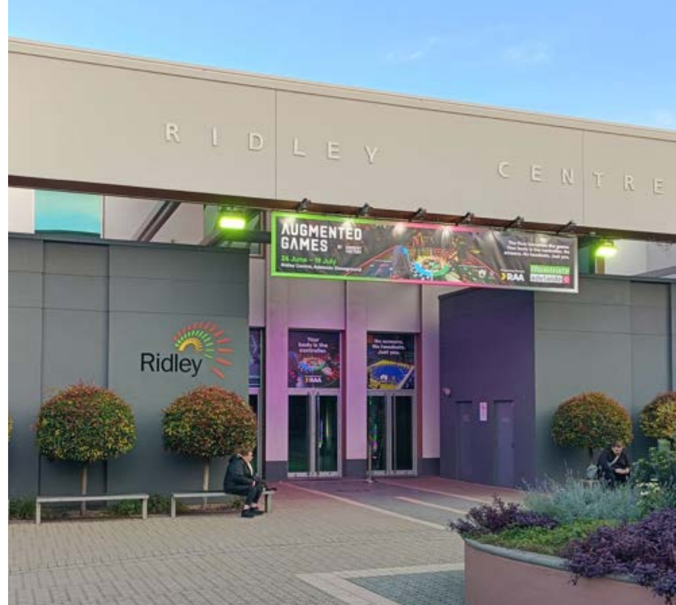
Alt Text: The image shows the entrance of Ridley Centre, featuring modern architecture with large glass doors and bright signage. A person sits on the bench outside.
